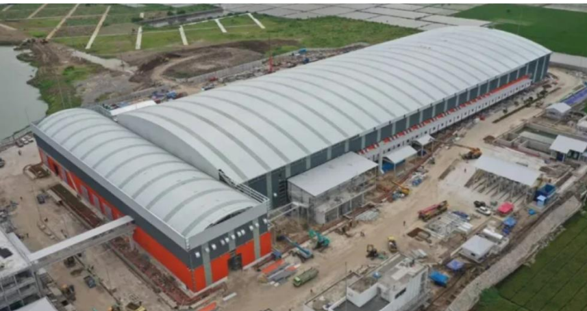
Gambar 2.11 RDF Plant Rorotan
